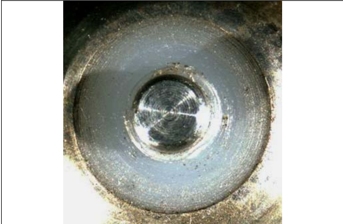
Photo 4: Condition of the main seat after testing on test article TA-1A.
